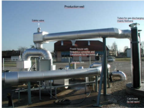
Figure 13, Geothermal system (doublet) in the Austrian town of Altheim, showing its main components, other than district heating piping, source: G. Pernecker, presentation of the project at the Calgary conference [28] 44
