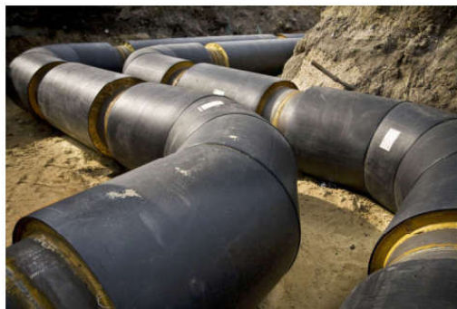
Figure 15, Usual size of the piping within the geothermal system based on hot water, Iceland, www.verkis.is , presentation by T. Johannesson at Cornell, 2016
